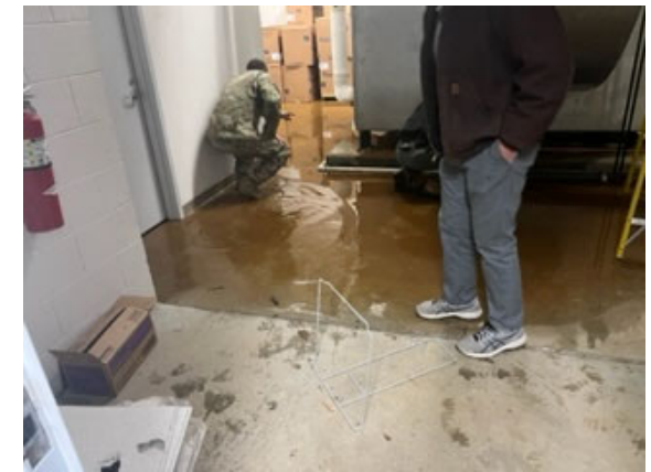
Elliot Storm Damage - Emergent
